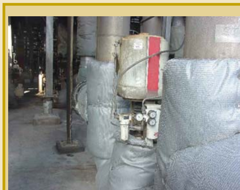
After installation of piping complete.
